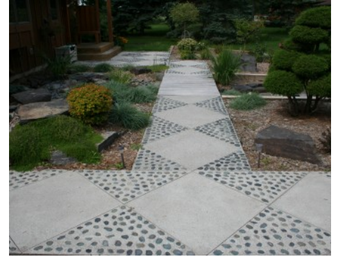
Private Residence - Walkway - Bomanite Revealed Diamond Shape
