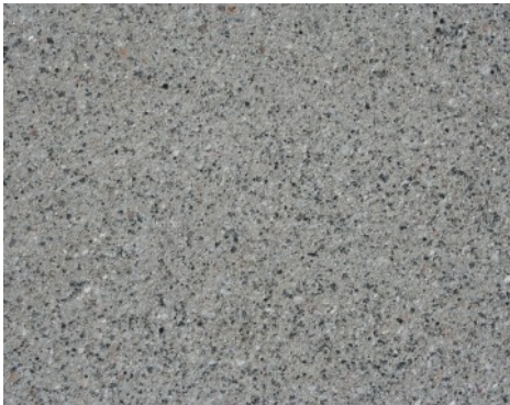
Private Residence - Walkway - Bomanite Revealed Close Up
