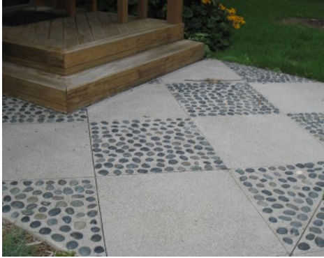
Private Residence - Walkway - Bomanite Revealed With Beach Pebble Embeds
