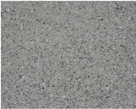
Private Residence - Walkway - Bomanite Revealed Close Up
