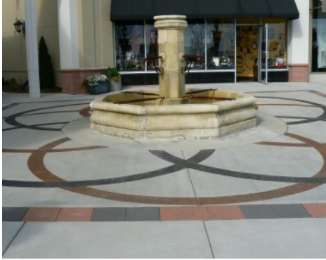
The Summit Shopping Center Plaza - Bomanite Chemical Stain
