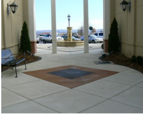
The Summit Shopping Center Plaza - Bomanite Chemical Stain
