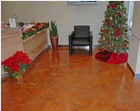
Bomanite Toppings Systems - Micro-Top with Patene Arectura Chemical Stain Interior Office Floor
