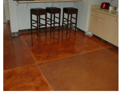
Bomanite Toppings Systems - Micro-Top with Patene Arectura Chemical Stain Interior Office Floor
