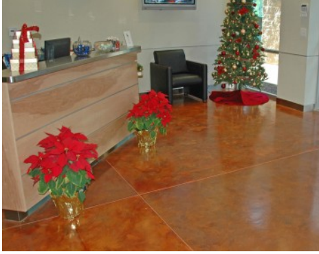
Bomanite Toppings Systems - Micro-Top with Patene Arectura Chemical Stain Interior Office Floor
