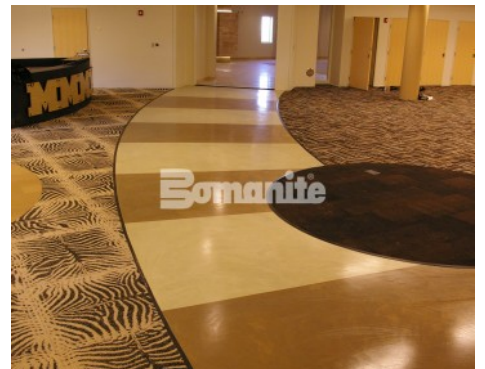
University of Missouri Brady Commons - Bomanite Micro-Top Interior Flooring
