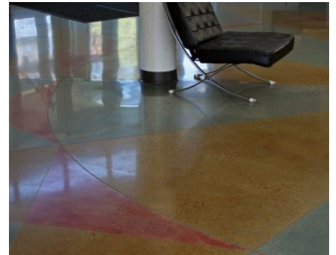
East Phillips Community Center - Bomanite Patene Teres Polished Concrete Floor
