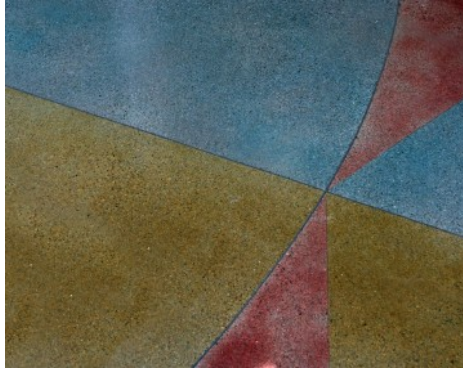
East Phillips Community Center - Bomanite Patene Teres Polished Concrete Floor
