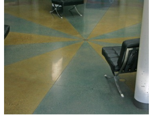
East Phillips Community Center - Bomanite Patene Teres Polished Concrete Floor
