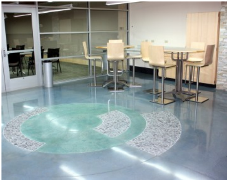
Wyoming Combined Labs - Polished Concrete Dye Patene Teres System
