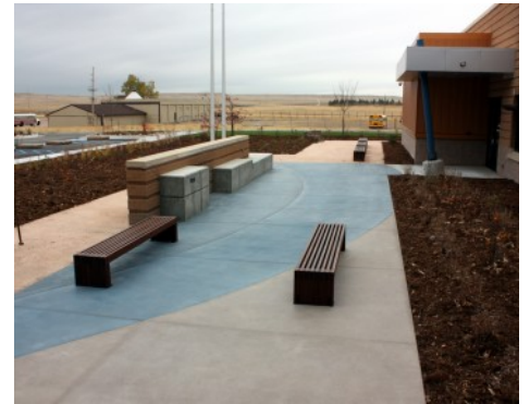
Wyoming Combined Labs - Exterior Sandscape Walkway
