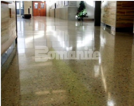
Army National Guard Windsor Colorado - Bomanite Patène Teres Polished Concrete Interior Floor
