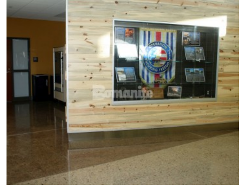
Army National Guard Windsor Colorado - Bomanite Patène Teres Polished Concrete Interior Floor
