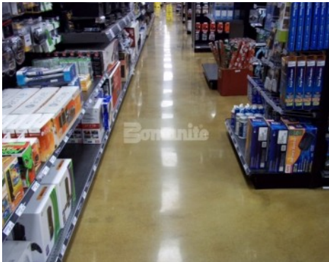
Hanscom MA Airforce Base PX - Bomanite Patene Teres Custom Polished Interior Floor
