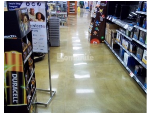
Hanscom MA Airforce Base PX - Bomanite Patene Teres Custom Polished Interior Floor
