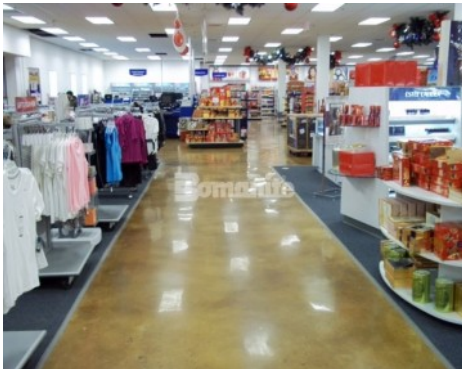
Fort Hamilton New York PX - Interior Floor with the Bomanite Custom Polishing Patene Teres System with Concrete Dye
