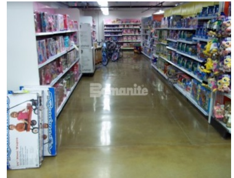
Fort Hamilton New York PX - Interior Floor with the Bomanite Custom Polishing Patene Teres System with Concrete Dye
