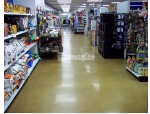
Fort Hamilton New York PX - Interior Floor with the Bomanite Custom Polishing Patene Teres System with Concrete Dye
