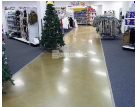
Fort Hamilton New York PX - Interior Floor with the Bomanite Custom Polishing Patene Teres System with Concrete Dye
