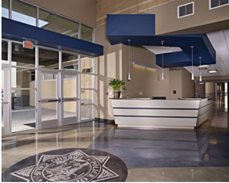
Fresno Police Facility - Regional Training Center - Bomanite Patene Teres Concrete Dye Polished Floor
