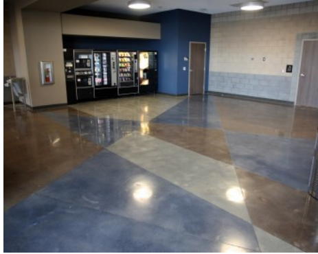
Fresno Police Facility - Regional Training Center - Bomanite Patene Teres Concrete Dye Polished Floor
