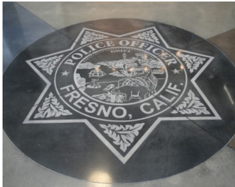
Fresno Police Facility - Regional Training Center - Bomanite Patene Teres Concrete Dye Polished Floor
