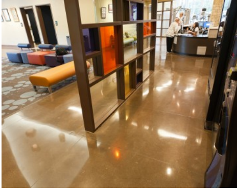
Heights Rec Center - Bomanite Renaissance - Integrally colored polished concrete
