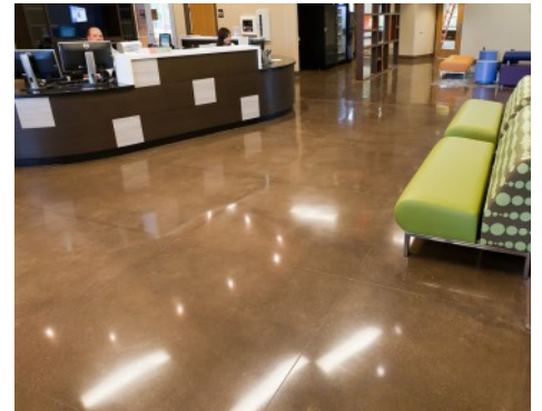
Heights Rec Center - Bomanite Renaissance - Integrally colored polished concrete
