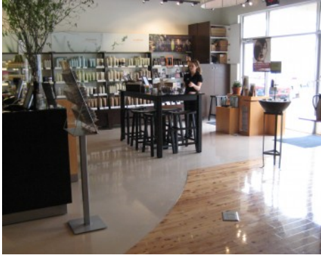
Aveda Salon - Bomanite Custom Polishing System Modena
