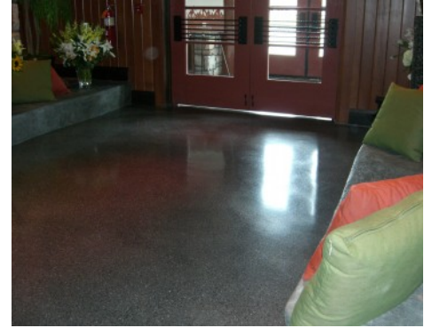
RedStone American Grill - Bomanite Modena Polished Concrete
