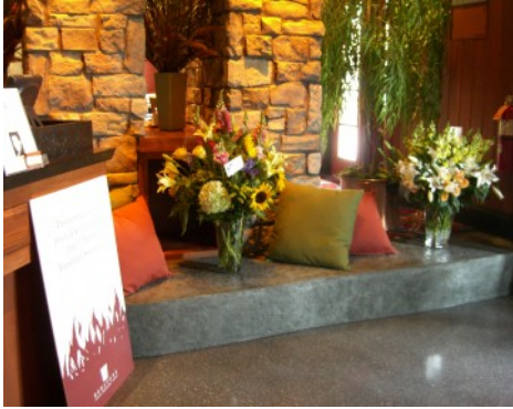
RedStone American Grill - Bomanite Modena Polished Concrete
