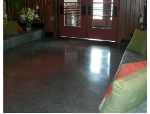
RedStone American Grill - Bomanite Modena Polished Concrete
