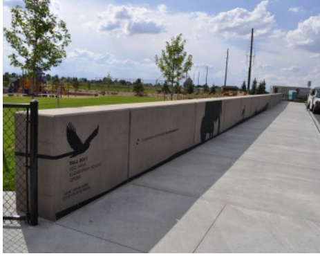
St. Vrain Elementary School - Sandstone Texture Interpretive Wall
