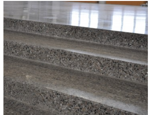
St. Vrain Elementary School - Custom Polished Concrete Gym Steps
