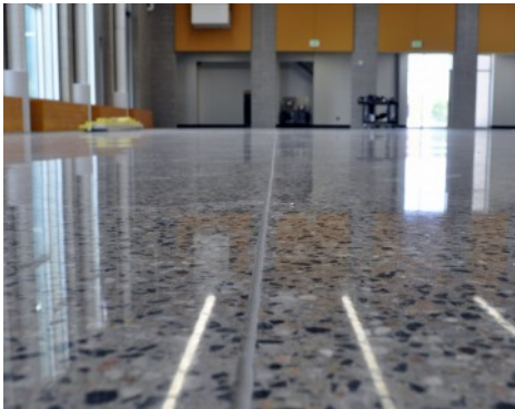
St. Vrain Elementary School - Custom Polished Concrete in Cafeteria
