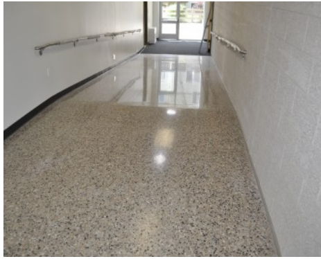
St. Vrain Elementary School - Polished Concrete Hallway Ramp
