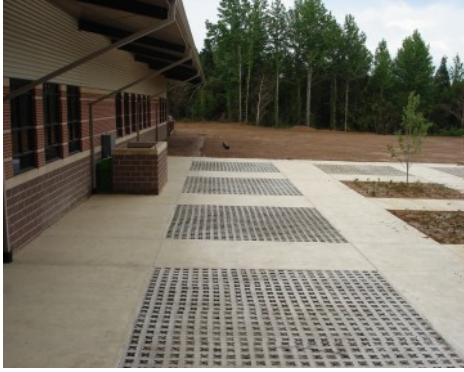
Wooster Elementary School - Grasscrete Partially Concealed System with Bomanite Imprinted Concrete
