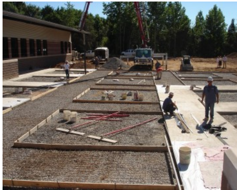
Wooster Elementary School - Grasscrete Edge Forming and Prep
