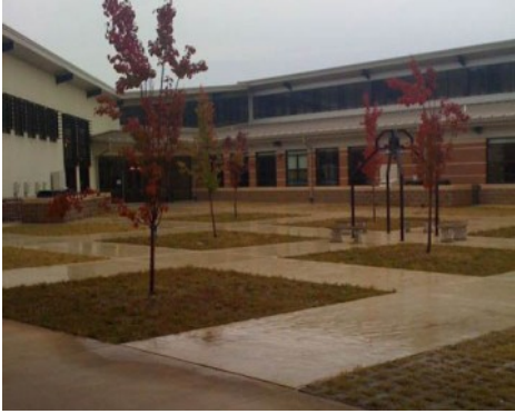
Wooster Elementary School - Finished landscaping with Partially Concealed Grasscrete System
