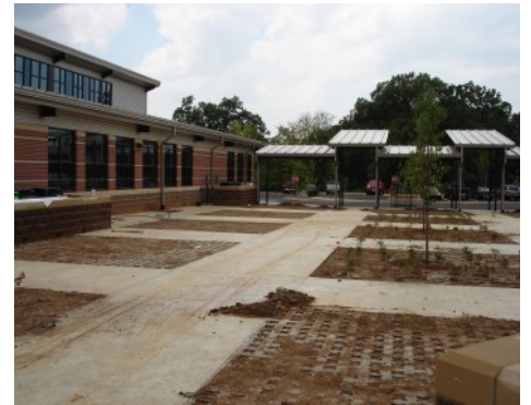
Wooster Elementary School - Grasscrete Voids being filled with soil and seed
