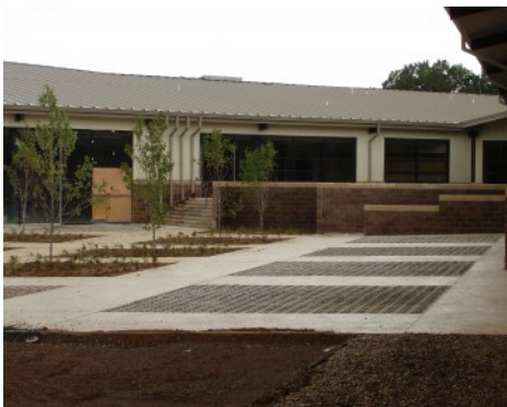
Wooster Elementary School - Grasscrete and Bomanite Imprinted Concrete
