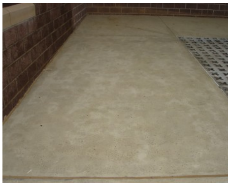
Wooster Elementary School - Grasscrete with Bomanite Imprinted Concrete - Coquina Texture
