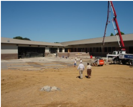
Wooster Elementary School - Grasscrete Sub Base Prep
