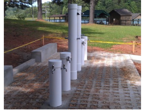
Camp Bud Schiele - Cub Scout Rinse Station - Stone Filled Grasscrete System Finished Installation
