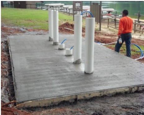
Camp Bud Schiele - Cub Scout Rinse Station - Concrete Pour
