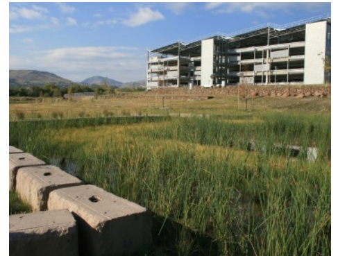
NREL Detention Pond - Partially Concealed Grasscrete System
