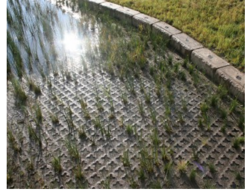
NREL Detention Pond - Partially Concealed Grasscrete System
