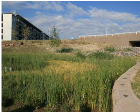
NREL Detention Pond - Partially Concealed Grasscrete System
