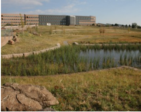
NREL Detention Pond - Partially Concealed Grasscrete System
