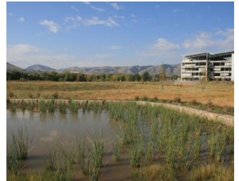
NREL Detention Pond - Partially Concealed Grasscrete System
