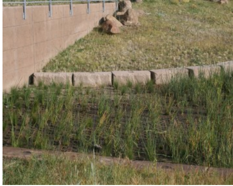
NREL Detention Pond - Partially Concealed Grasscrete System
