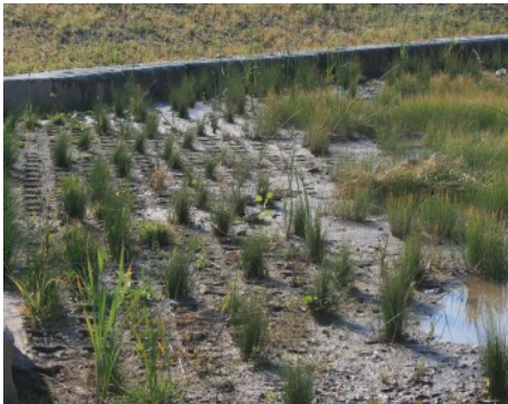
NREL Detention Pond - Partially Concealed Grasscrete System
