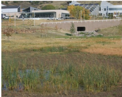
NREL Detention Pond - Partially Concealed Grasscrete System
