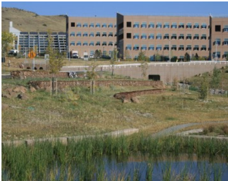
NREL Detention Pond - Partially Concealed Grasscrete System
