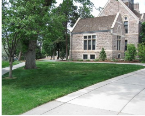
Colorado College - Emergency Vehicle Access Concealed Grasscrete System
