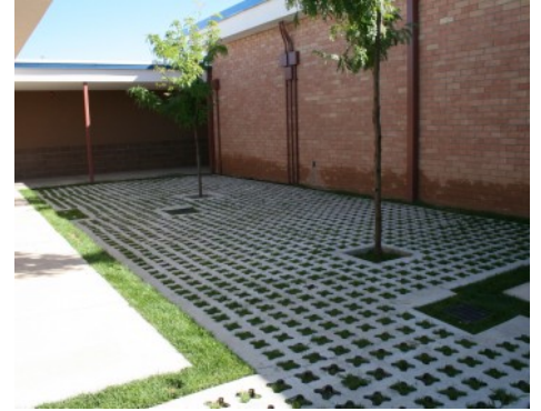
St. Mikes School - Entry Courtyard - Grasscrete Partially Concealed System For Stormwater Runoff
