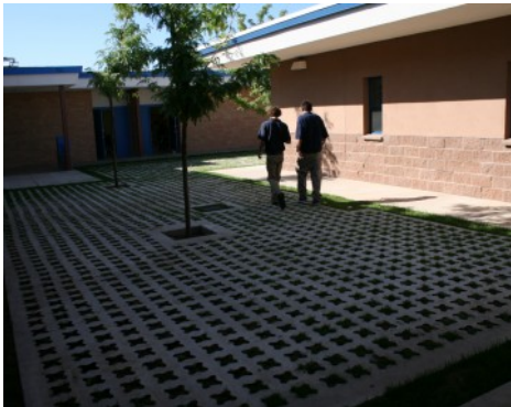
St. Mikes School - Entry Courtyard - Grasscrete Partially Concealed System For Heavy Foot Traffic
