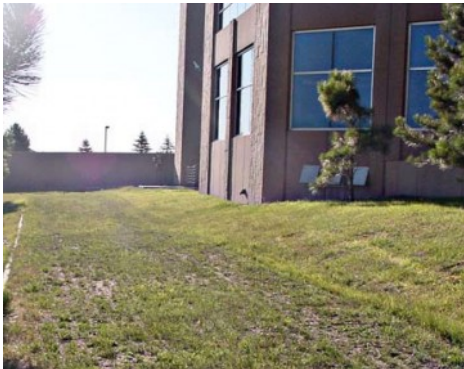
Corporate Express Office Building - Utility Vehicle Access
