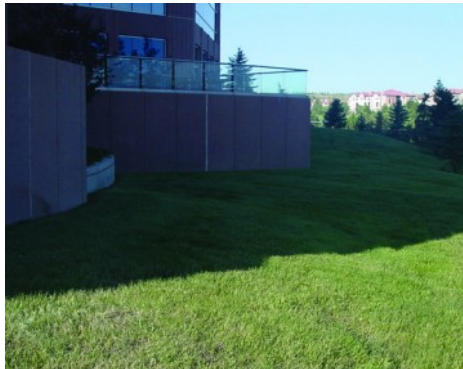
Corporate Express Office Building - Utility Vehicle Access
