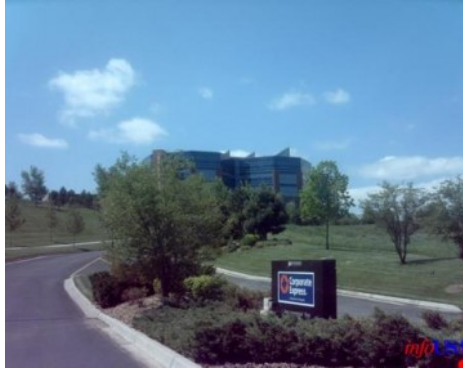
Corporate Express Office Building - Utility Vehicle Access
