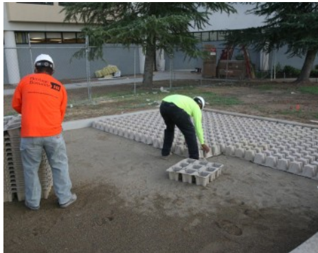
Clovis Community Hospital - Molded Pulp Former Installation
