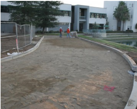
Clovis Community Hospital - Molded Pulp Former Installation
