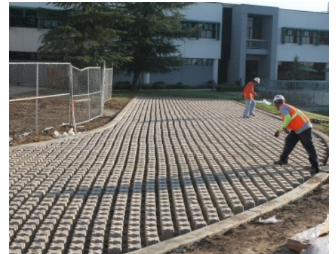
Clovis Community Hospital - Molded Pulp Former Installation
