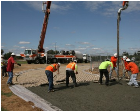
Clovis Community Hospital - Concrete Pour Process
