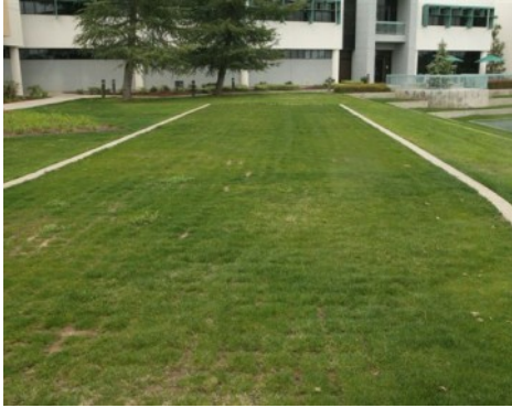
Clovis Community Hospital - Emergency Vehicle Access Grasscrete Concealed System - Final Installation
