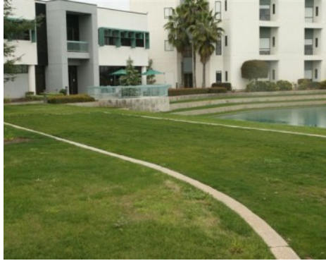
Clovis Community Hospital - Grasscrete Concealed System - Final Installation
