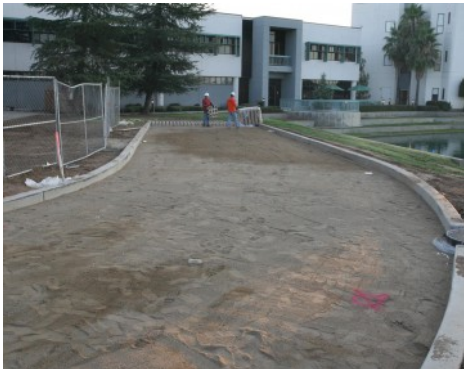
Clovis Community Hospital - Molded Pulp Former Installation
