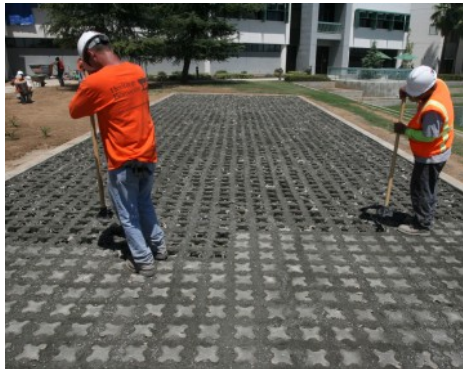
Clovis Community Hospital - Opening Molded Pulp Former Voids
