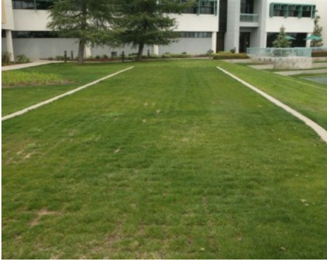
Clovis Community Hospital - Emergency Vehicle Access Grasscrete Concealed System - Final Installation
