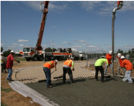
Clovis Community Hospital - Concrete Pour Process
