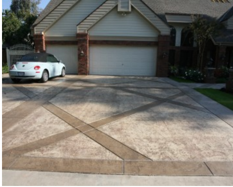
Bomanite Imprinted Concrete - Residential Driveway - Slate Texture
