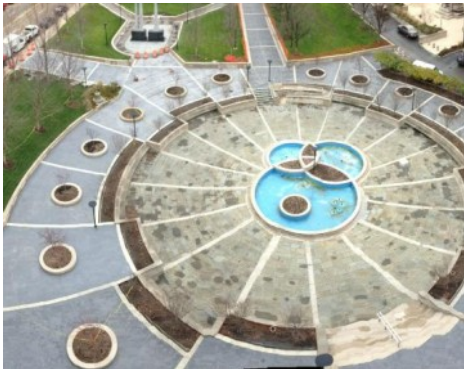
Peoria Courthouse Plaza Renovation - Imprint Systems English Slate Texture
