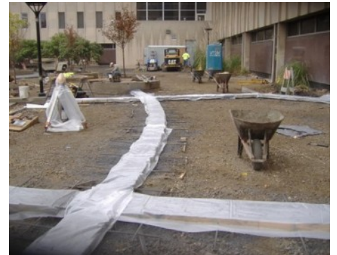
Peoria Courthouse Plaza Renovation - Before
