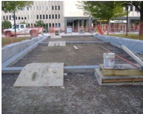
Peoria Courthouse Plaza Renovation - Before
