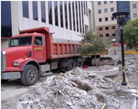
Peoria Courthouse Plaza Renovation - Before
