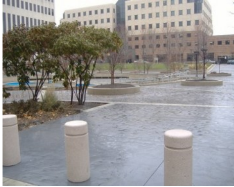
Peoria Courthouse Plaza Renovation - Imprint Systems English Slate Texture
