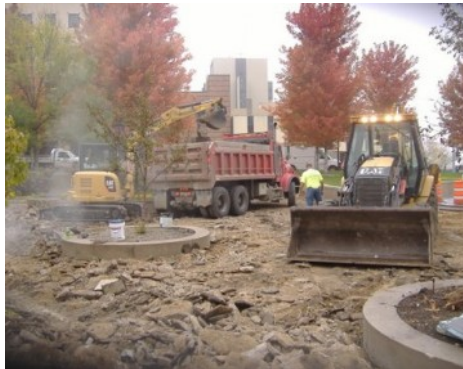
Peoria Courthouse Plaza Renovation - Before
