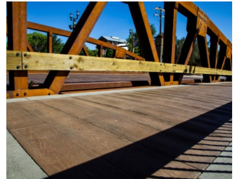
Temecula Bridge - Bomanite Imprint Systems Boardwalk Pattern
