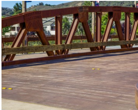
Temecula Bridge - Bomanite Imprint Systems Boardwalk Pattern
