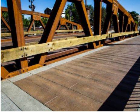
Temecula Bridge - Bomanite Imprint Systems Boardwalk Pattern
