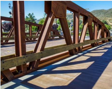
Temecula Bridge - Bomanite Imprint Systems Boardwalk Pattern
