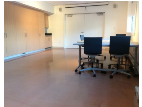
Deerfield Academy - Bomanite Modena SL Custom Polished Concrete
