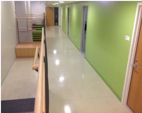
Deerfield Academy - Bomanite Modena SL Custom Polished Concrete
