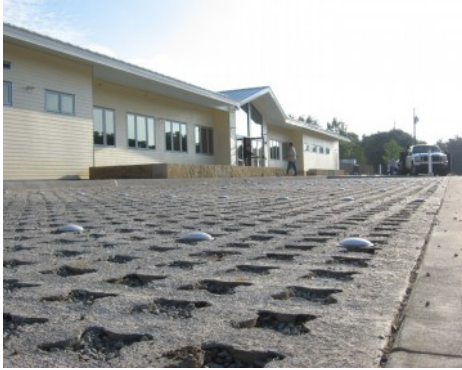
Grasscrete Parking Lot Finished Installation
