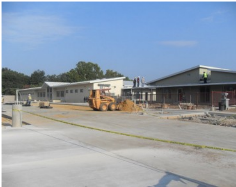
Grasscrete Sub Base Prep for Former installation
