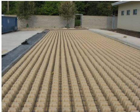
Grasscrete Molded Pulp Formers Installed
