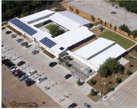
Grasscrete Parking Lot Finished Installation
