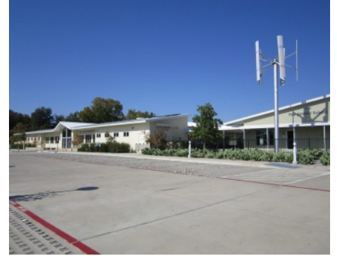
Grasscrete Parking Lot Finished Installation
