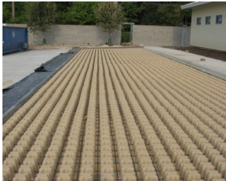
Grasscrete Molded Pulp Formers Installed
