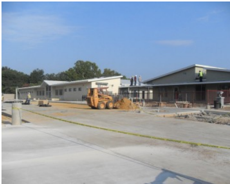
Grasscrete Sub Base Prep for Former installation
