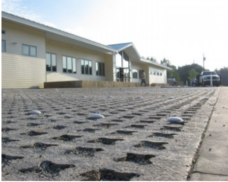
Grasscrete Parking Lot Finished Installation
