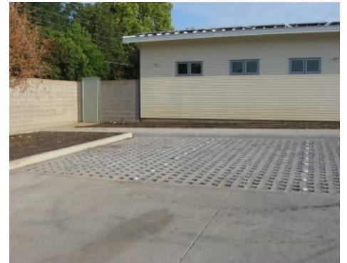
Grasscrete Parking Lot Finished Installation
