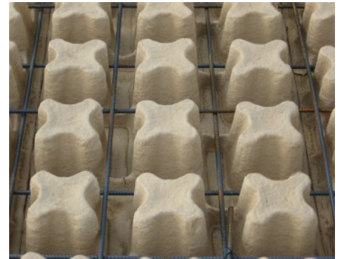
Grasscrete Molded Pulp Formers with Rebar
