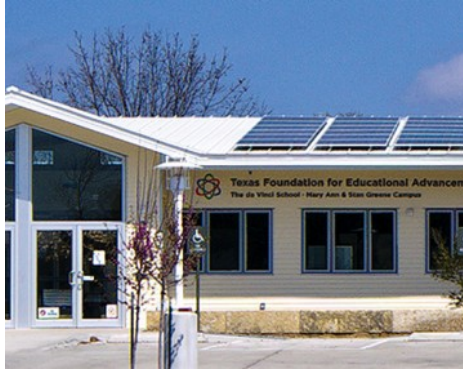
Grasscrete Parking Lot Finished Installation
