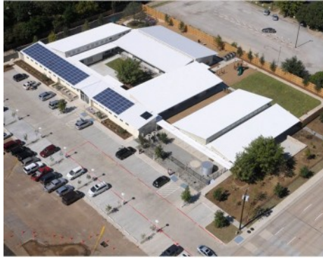
Grasscrete Parking Lot Finished Installation
