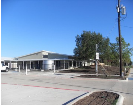
Grasscrete Parking Lot Finished Installation
