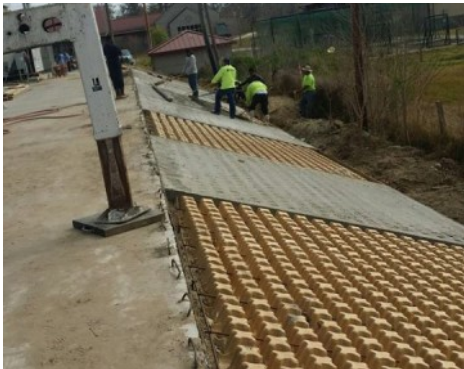
Jean LaFitte Auditorium - Grasscrete Installation Voids Removed
