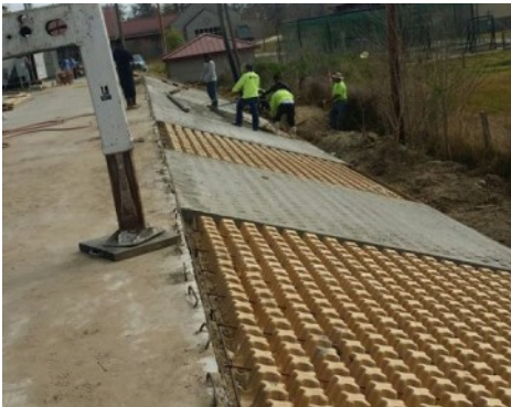
Jean LaFitte Auditorium - Grasscrete Installation Voids Removed
