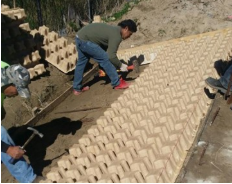
Jean LaFitte Auditorium - Grasscrete Molded Pulp Former Installation
