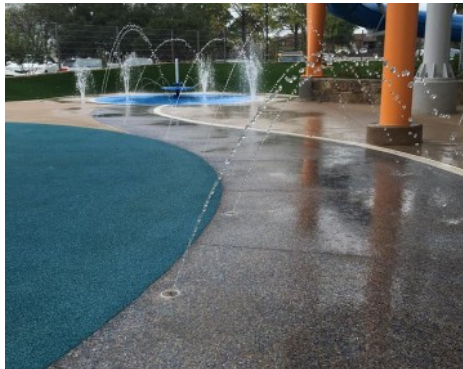
Tandy Family YMCA - Bomanite Revealed and Bomanite Sandstone Texture Splashpark
