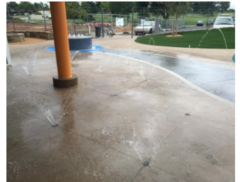
Tandy Family YMCA - Bomanite Revealed and Bomanite Sandstone Texture Splashpark
