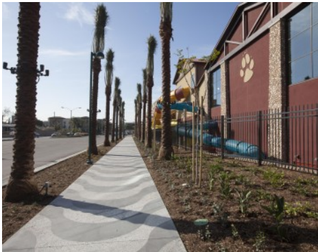
Great Wolf Lodge Resort - Bomanite Imprint Systems - Alicante Pattern with Bomanite Alloy Finish
