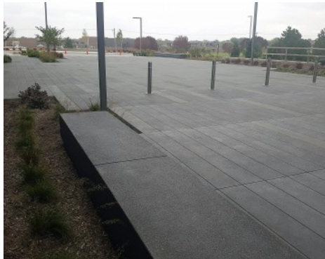
Garmin Expansion - Bomanite Sandstone Texture with Bomanite Con-Color
