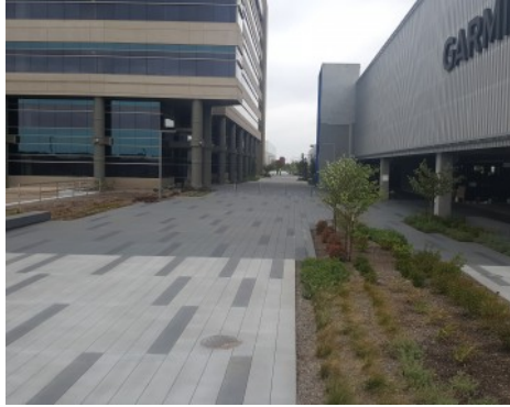
Garmin Expansion - Bomanite Sandstone Texture with Bomanite Con-Color
