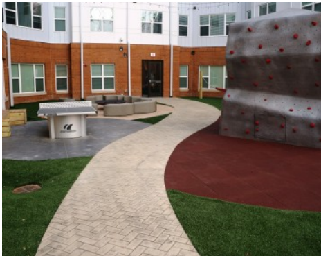
Bomanite Imprinted Concrete Systems - Bomacron Herringbone Used Brick and Bomacron Running Bond Used Brick
