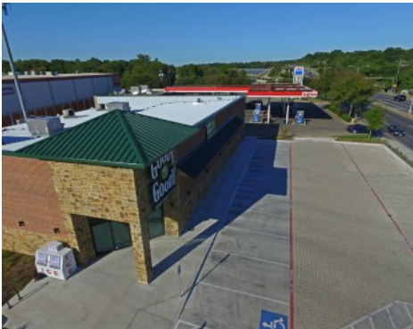
Goody Goody Liquor Store Parking Lot - Bomanite Pervious Grasscrete Stone Filled System - ADA Access
