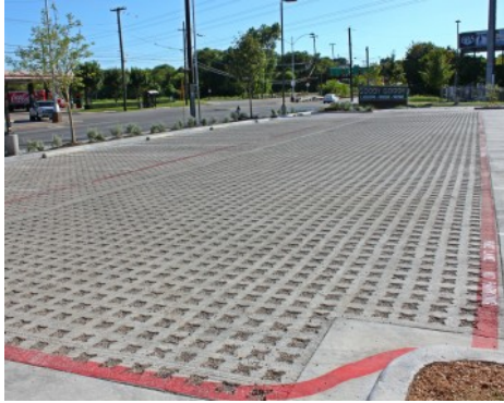
Goody Goody Liquor Store Parking Lot - Bomanite Pervious Grasscrete Stone Filled System - ADA Access
