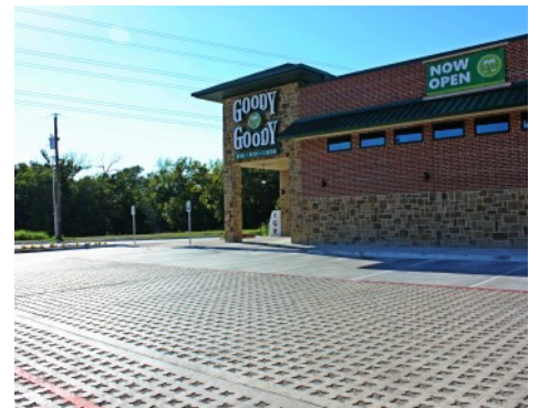
Goody Goody Liquor Store Parking Lot - Bomanite Pervious Grasscrete Stone Filled System - ADA Access
