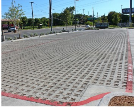
Goody Goody Liquor Store Parking Lot - Bomanite Pervious Grasscrete Stone Filled System - ADA Access
