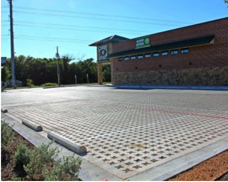
Goody Goody Liquor Store Parking Lot - Bomanite Pervious Grasscrete Stone Filled System - ADA Access
