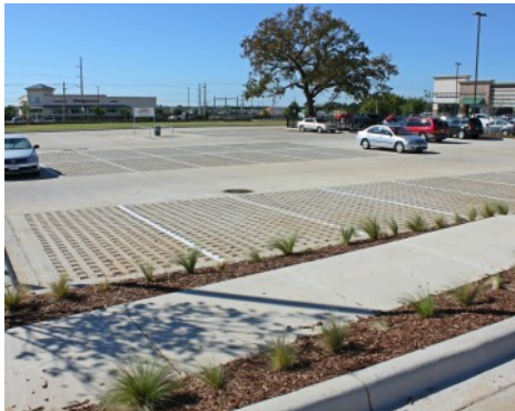
Sprouts Farmers Market Denton Tx - Bomanite Pervious Concrete Grasscrete Stone Filled System
