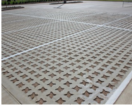
Sprouts Farmers Market Denton Tx - Bomanite Pervious Concrete Grasscrete Stone Filled System
