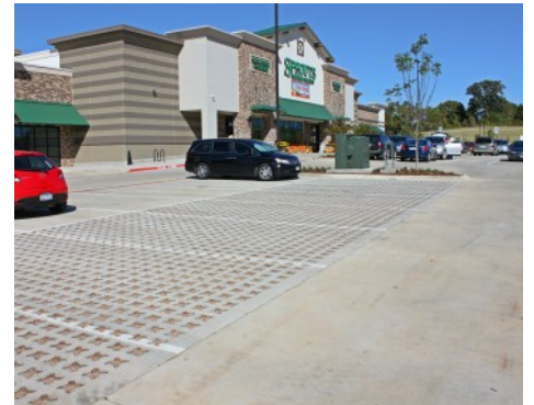
Sprouts Farmers Market Denton Tx - Bomanite Pervious Concrete Grasscrete Stone Filled System
