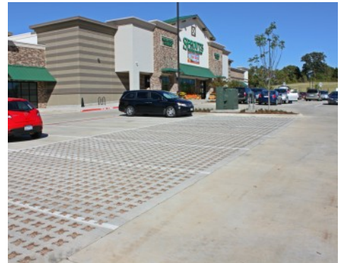
Sprouts Farmers Market Denton Tx - Bomanite Pervious Concrete Grasscrete Stone Filled System
