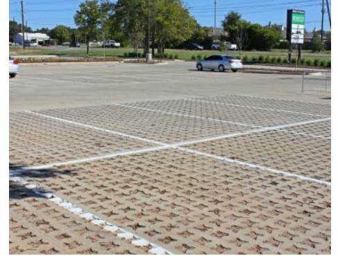
Sprouts Farmers Market Denton Tx - Bomanite Pervious Concrete Grasscrete Stone Filled System
