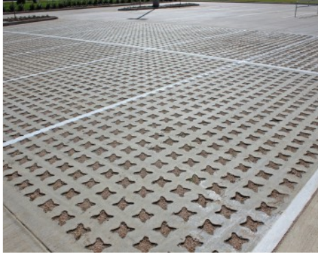
Sprouts Farmers Market Denton Tx - Bomanite Pervious Concrete Grasscrete Stone Filled System
