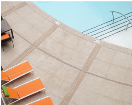
Hartford Commons The Edge Apartments - Bomanite Exposed Aggregate Alloy System Pool Deck
