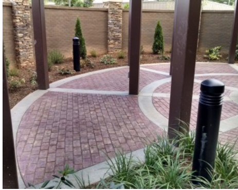
Marriott Courtyard Hotel Guest Terrace - Bomanite Imprint Systems - Running Bond Used Brick Pattern
