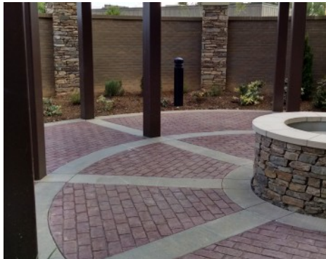
Marriott Courtyard Hotel Guest Terrace - Bomanite Imprint Systems - Running Bond Used Brick Pattern
