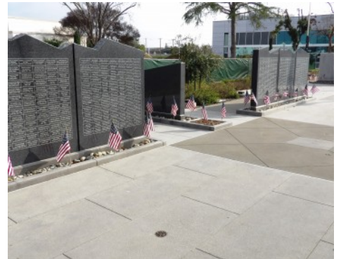
Veterans Walk of Honor - Bomanite Exposed Aggregate Sandscape Texture
