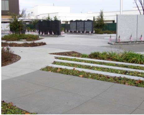
Veterans Walk of Honor - Bomanite Exposed Aggregate Sandscape Texture
