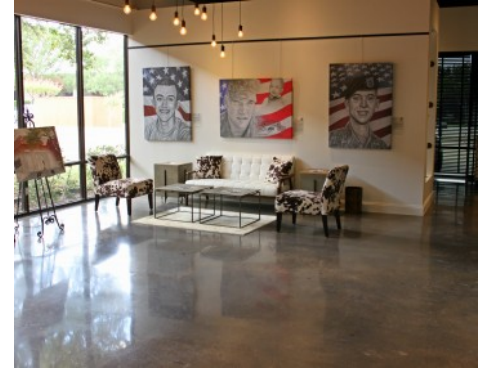
American Fallen Soldiers Gallery - Bomanite Concrete Dye Patene Teres Polished Concrete Floors
