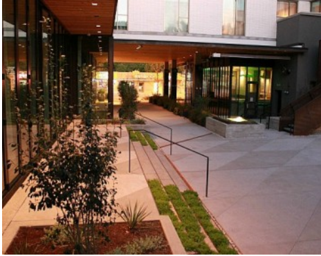
South Congress Hotel - Bomanite Exposed Aggregate Sandblast Finishes with concrete planter walls and water features
