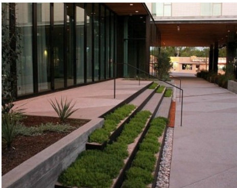
South Congress Hotel - Bomanite Exposed Aggregate Sandblast Finishes with concrete planter walls and water features
