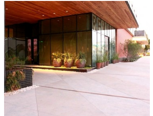
South Congress Hotel - Bomanite Exposed Aggregate Sandscape Texture and Sandblast Finishes with concrete planter walls and water features
