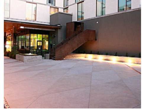
South Congress Hotel - Bomanite Exposed Aggregate Sandblast Finishes with concrete planter walls and water features
