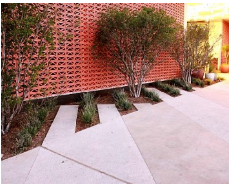
South Congress Hotel - Bomanite Exposed Aggregate Sandscape Texture and Sandblast Finishes with concrete planter walls and water features
