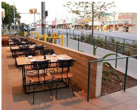
South Congress Hotel - Bomanite Exposed Aggregate Sandscape Texture and Sandblast Finishes with concrete planter walls and water features
