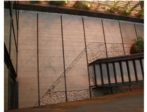
South Congress Hotel - Bomanite Exposed Aggregate Sandscape Texture and Sandblast Finishes with concrete planter walls and water features
