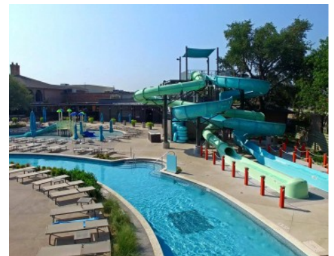
Hilton Anatole Hotel Jade Waters Pool Complex - Bomanite Exposed Aggregate Sandscape Texture and Sandscape Refined with Bomanite Shifting Sands Erosion Series Imprinted Concrete
