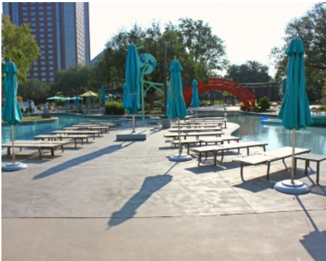
Hilton Anatole Hotel Jade Waters Pool Complex - Bomanite Exposed Aggregate Sandstone Texture and Sandstone Refined with Bomanite Shifting Sands Erosion Series Imprinted Concrete
