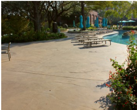
Hilton Anatole Hotel Jade Waters Pool Complex - Bomanite Exposed Aggregate Sandstone Texture and Sandstone Refined with Bomanite Shifting Sands Erosion Series Imprinted Concrete
