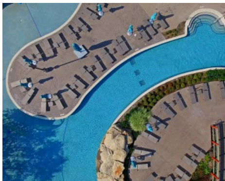
Hilton Anatole Hotel Jade Waters Pool Complex - Bomanite Exposed Aggregate Sandscape Texture and Sandscape Refined with Bomanite Shifting Sands Erosion Series Imprinted Concrete
