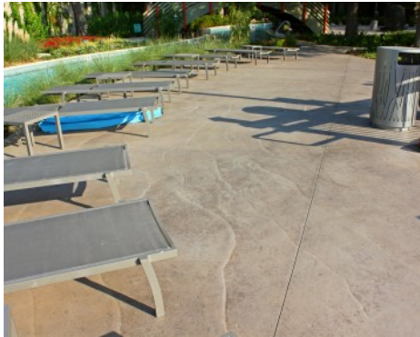
Hilton Anatole Hotel Jade Waters Pool Complex - Bomanite Exposed Aggregate Sandstone Texture and Sandstone Refined with Bomanite Shifting Sands Erosion Series Imprinted Concrete
