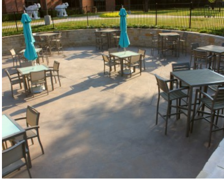
Hilton Anatole Hotel Jade Waters Pool Complex - Bomanite Exposed Aggregate Sandstone Texture and Sandstone Refined with Bomanite Shifting Sands Erosion Series Imprinted Concrete
