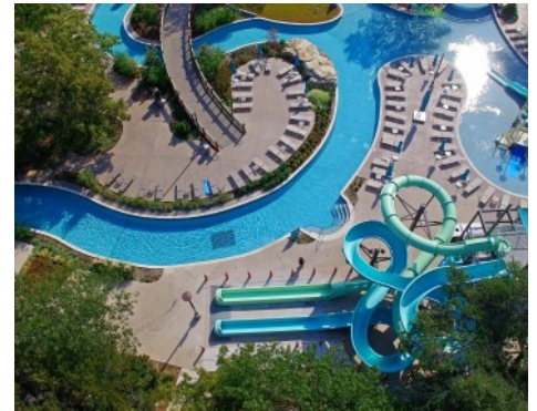
Hilton Anatole Hotel Jade Waters Pool Complex - Bomanite Exposed Aggregate Sandscape Texture and Sandscape Refined with Bomanite Shifting Sands Erosion Series Imprinted Concrete
