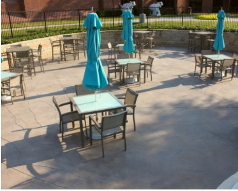
Hilton Anatole Hotel Jade Waters Pool Complex - Bomanite Exposed Aggregate Sandstone Texture and Sandstone Refined with Bomanite Shifting Sands Erosion Series Imprinted Concrete
