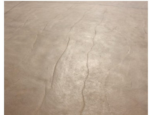
Hilton Anatole Hotel Jade Waters Pool Complex - Bomanite Exposed Aggregate Sandstone Texture and Sandstone Refined with Bomanite Shifting Sands Erosion Series Imprinted Concrete
