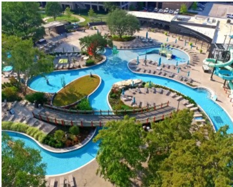
Hilton Anatole Hotel Jade Waters Pool Complex - Bomanite Exposed Aggregate Sandscape Texture and Sandscape Refined with Bomanite Shifting Sands Erosion Series Imprinted Concrete
