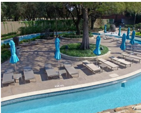
Hilton Anatole Hotel Jade Waters Pool Complex - Bomanite Exposed Aggregate Sandscape Texture and Sandscape Refined with Bomanite Shifting Sands Erosion Series Imprinted Concrete
