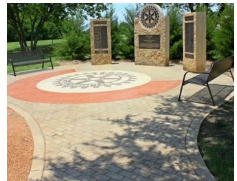
Mesquite Rotary Club Grove of Honor Memorial - Bomanite Imprint Systems Running Bond Used Brick Walkway with Exposed Aggregate Sandscape Refined System Logo
