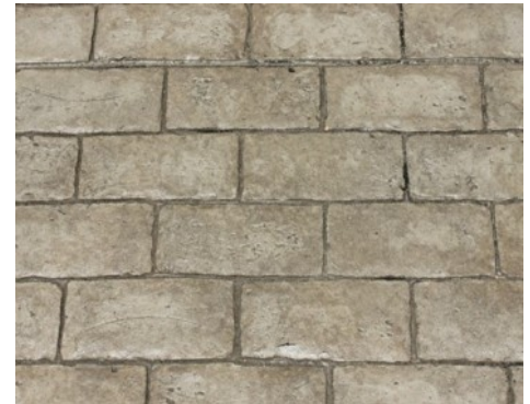
Mesquite Rotary Club Grove of Honor Memorial - Bomanite Imprint Systems Running Bond Used Brick Walkway (close up) with Exposed Aggregate Sandstone Refined System Logo
