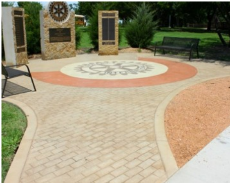
Mesquite Rotary Club Grove of Honor Memorial - Bomanite Imprint Systems Running Bond Used Brick Walkway with Exposed Aggregate Sandscape Refined System Logo
