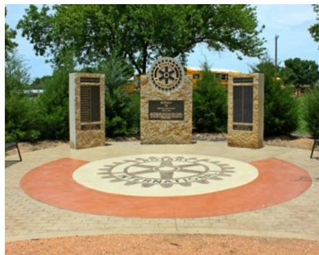
Mesquite Rotary Club Grove of Honor Memorial - Bomanite Imprint Systems Running Bond Used Brick Walkway with Exposed Aggregate Sandstone Refined System Logo
