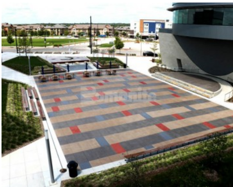
Lenexa Civic Center Plaza; Bomanite Exposed Aggregate Sandscape Texture System with Bomanite Con-Color
