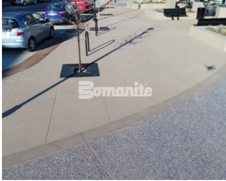
DELO - Downtown East Louisville: Exposed Aggregate Sandscape Texture Streetscape; Sandscape Refined Seat Walls
