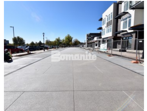
DELO - Downtown East Louisville: Exposed Aggregate Sandscape Texture Streetscape; Sandscape Refined Seat Walls
