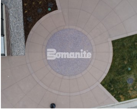
DELO - Downtown East Louisville: Exposed Aggregate Sandscape Texture Streetscape; Sandscape Refined Seat Walls
