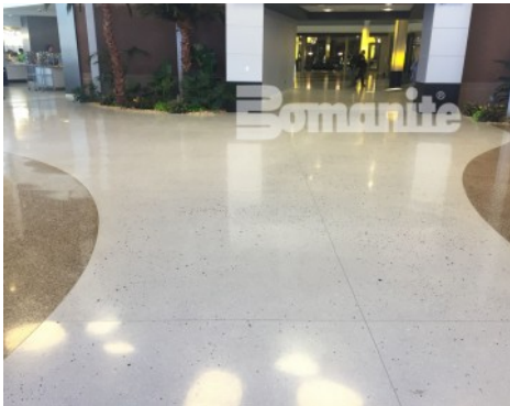
Infinite Campus Cafeteria - Bomanite Custom Polished Systems; Modena Monolithic and Renaissance Deep Grind
