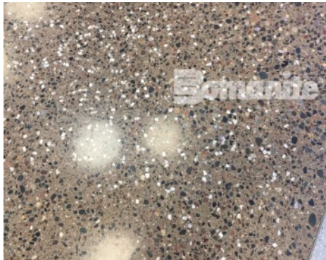
Infinite Campus Cafeteria - Bomanite Custom Polished Systems; Renaissance Deep Grind Close Up
