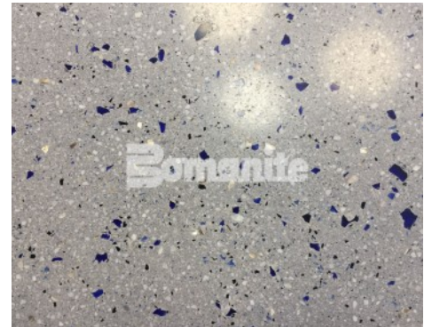
Infinite Campus Cafeteria - Bomanite Custom Polished Systems; Modena Monolithic Close Up
