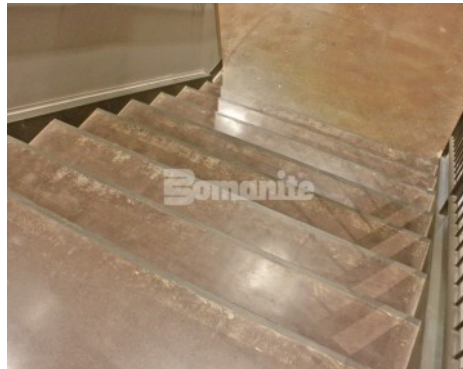
Hope Fellowship Church - Bomanite Custom Polishing Patene Teres System Interior Floor
