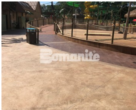
Canobie Lake Park, Castaway Island Expansion by Harrington Bomanite installation of the Walkway and Plaza Stamped with Bomanite 11.5" Boardwalk Pattern and Regular Slate Textured Decorative Concrete
