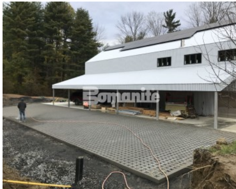
Voids Created, Final Finishing
