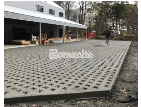
Voids Created, Final Finishing
