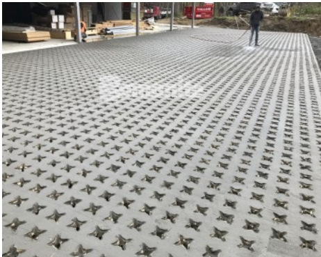
Voids Created, Final Finishing
