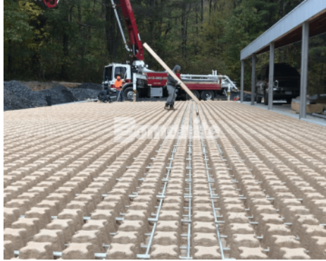
Laying of Molded Pulp Formers with Rebar
