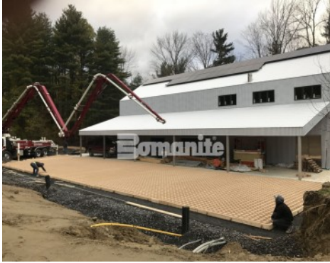
Laying of Molded Pulp Formers
