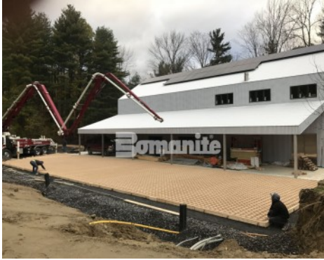
Laying of Molded Pulp Formers
