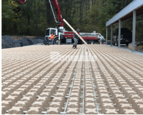
Laying of Molded Pulp Formers with Rebar
