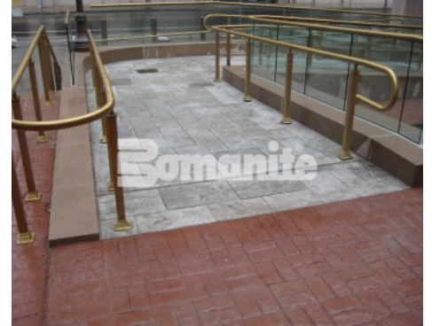
Tower Plaza - Bomanite Imprint Systems; Bomanite Basketweave Brick (no Texture) and Bomacron Medium Ashlar Slate
