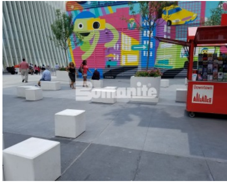
World Trade Center New York Tower 2 Street Design - Bomanite Alloy Exposed Aggregate System
