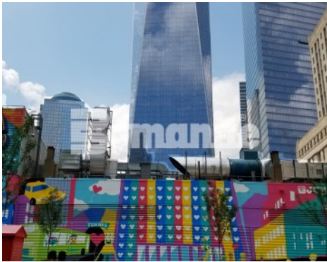
World Trade Center New York Tower 2 Street Design - Bomanite Alloy Exposed Aggregate System
