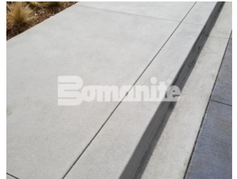
50 Fifty DTC Building - Denver, CO - Bomanite Exposed Aggregate Sandstone Refined System Walkways and Curbs
