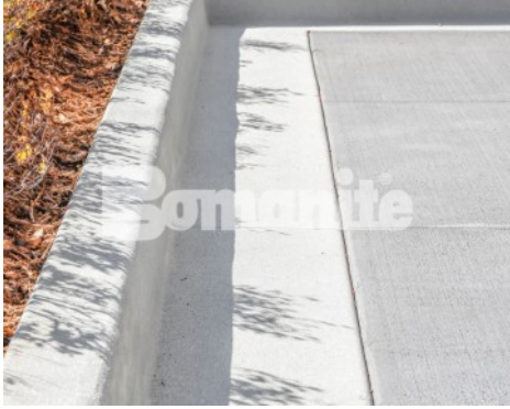
50 Fifty DTC Building - Denver, CO - Bomanite Exposed Aggregate Sandstone Refined System Walkways and Curbs
