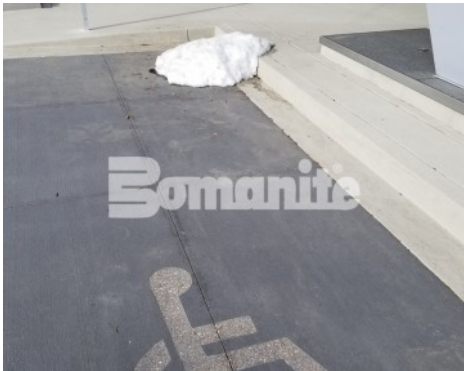
50 Fifty DTC Building - Denver, CO - Bomanite Exposed Aggregate Sandstone Refined System Walkways and Curbs
