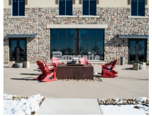
Gaylord Rockies Resort Colorado - Bomanite Exposed Aggregate Sandstone Texture Patio
