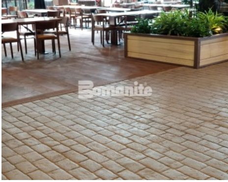
Gaylord Rockies Resort Colorado - Bomanite Imprint Systems
