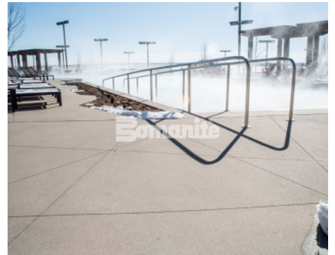
Gaylord Rockies Resort Colorado - Bomanite Exposed Aggregate Sandstone Texture Pool Deck
